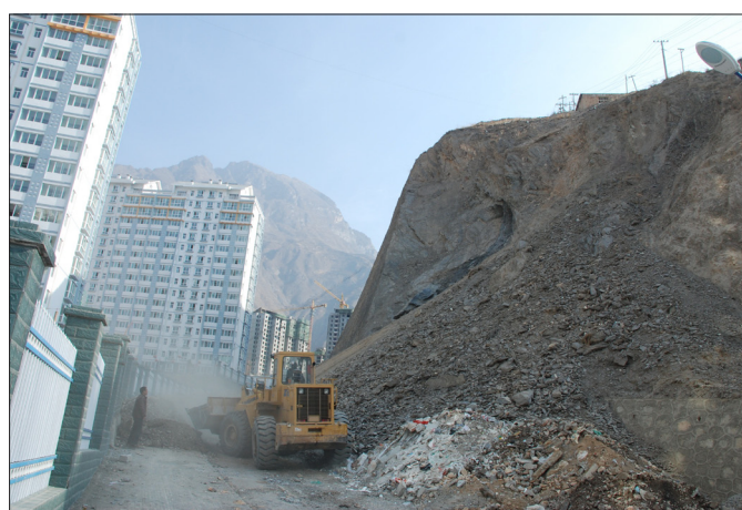
Figure 2. The south side slope site.
