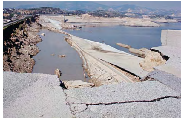
Figure 9 The failure of the upstream slope of the Lower San Fernando Dam shortly after the 1971 San Fernando earthquake. California narrowly avoided catastrophic flooding of 80 000 downstream homes. Liquefaction of the hydraulic fill caused loss of strength and slope instability, which left less than 1 m of free board after the earthquake. This picture shows the slide after emptying the reservoir; the paved road to the left indicates the former dam crest. Photograph by Leslie F. Harder, Jr.
