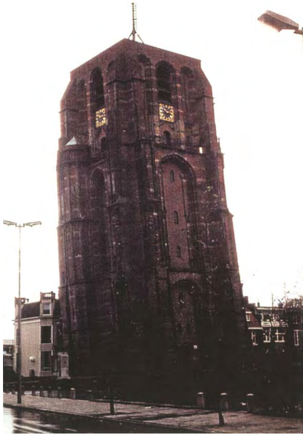
Figure 3 Leaning church tower due to differential settlement in soft Holocene sediments, a foundation problem near Lake IJssel, The Netherlands. de Mulder EFJ, Holland, International Union of Geological Sciences 'COGEOENVIRONMENT' photograph.
