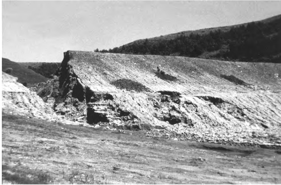
Figure 6 Failed earth dam constructed of dispersive soil, showing piping outlets on the downstream side, near Ramsgate, South Africa.
