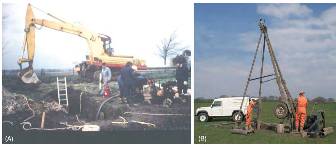
Figure 2 Two common methods of exploration. (A) The trial pit, with shoring and ladder for safe access and egress. (B) The percussion boring rig.
