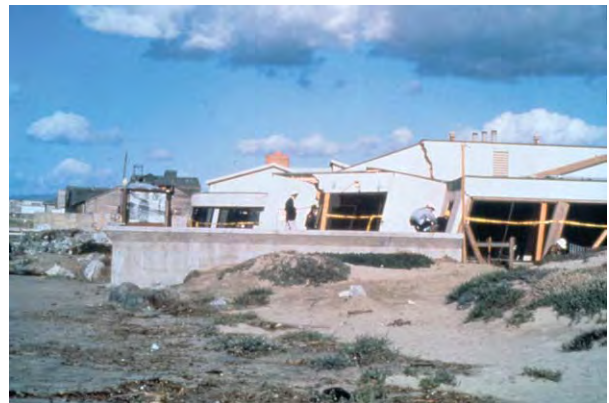
Figure 14 Damage to the Marine Laboratory at Moss Landing, Monterey Bay, California, during the 1989 magnitude 6.9 Loma Prieta earthquake. Lateral spreading caused the building pad foundations to spread apart. The laboratory was subsequently demolished. Photograph by Leslie F. Harder, Jr.
