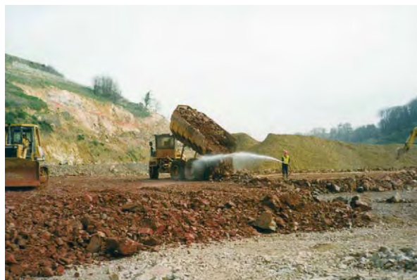
Figure 4 Watering rock fill during placement.
