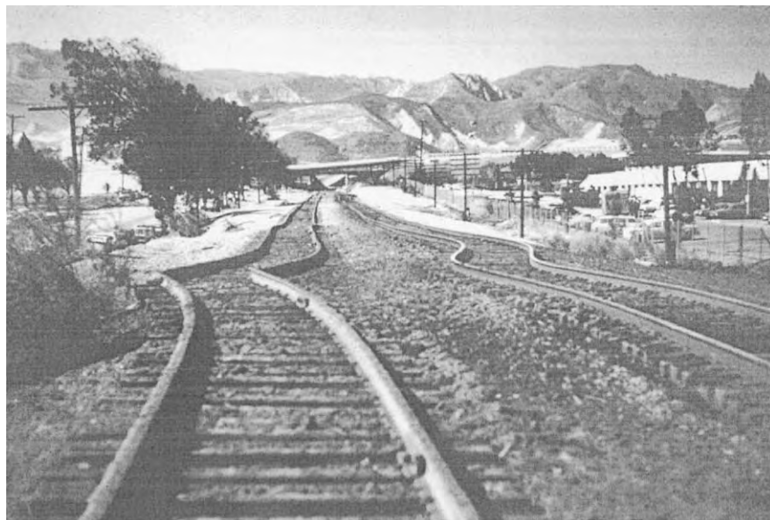
Figure 1 Engineering geological mapping records evidence of earthquake motion such as this railroad deformation indicating north to south shortening of the ground along the rail right of way. Most evidence of earthquake damage is fragile and likely to be destroyed by human activity within hours or days. (Photographed by Richard J. Proctor, then Chief Engineering Geologist, Metropolitan Water District of Southern California, at San Fernando Valley, California, February 1971.)
