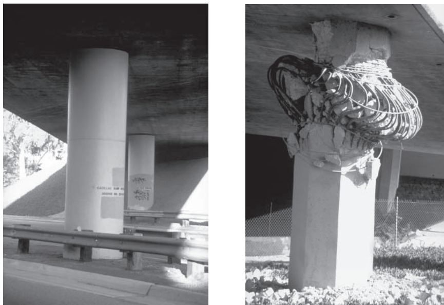
FIGURE 1.2 Comparison of retrofitted and unimproved concrete bridge columns following the 1994 Northridge, California, earthquake. Left: Cadillac Avenue ramp at Interstate 10 (Santa Monica Freeway). Right: Highway 118/Bull Creek Bridge. Reproduced courtesy of the National Information Service for Earthquake Engineering, University of California, Berkeley.
