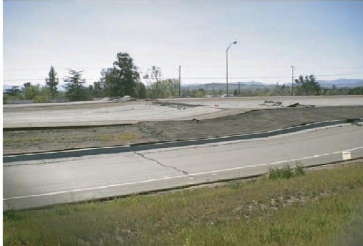
Figure 1. Settlement in a highway after the San Fernando earthquake, in 1971. (Courtesy of the National Information Service for Earthquake Engineering, EERC, University of California, Berkeley).
