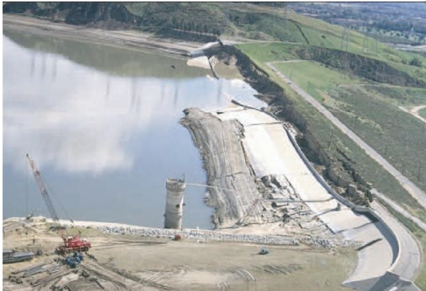
Figure 19. Lower San Fernando dam after the San Fernando earthquake (1971). (Courtesy of the National Information Service for Earthquake Engineering, EERC, University of California, Berkeley).
