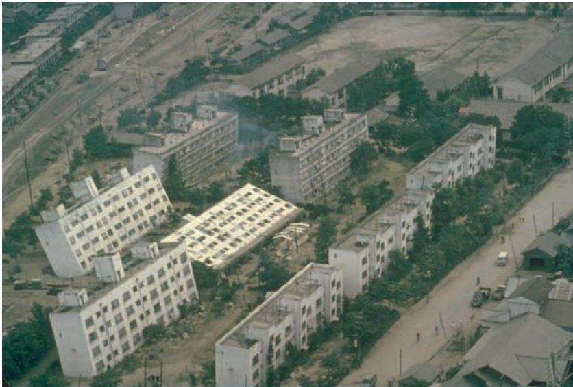
Figure 16. Liquefaction at buildings foundation, Niigata earthquake (1964). (Courtesy of the National Information Service for Earthquake Engineering, EERC, University of California, Berkeley).
