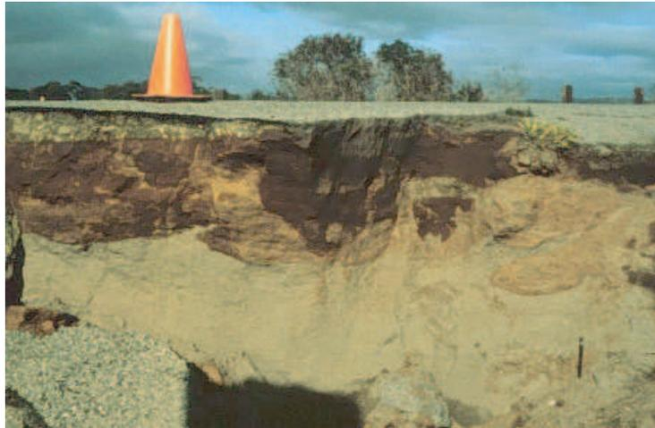
Figure 21. Detail of a failed road due to liquefaction after the Loma Prieta earthquake (1989); Moss Landing State Beach. (Photo: Dan Orange; Courtesy of Justin Revenaugh, Earth Sciences, University of California).
