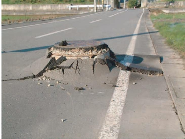
Figure 2. Settlement of a road surface after the Niigata 2004 earthquake (Courtesy of James Arendt, Japan).
