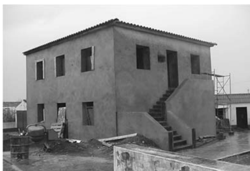
Fig. 19.38. House with finished plastering operation
