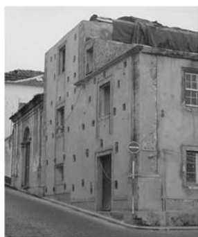
Fig. 19.37. Application of the reinforced plaster
