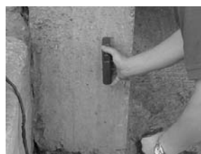
Fig. 19.21. Survey of bar arrangement using scanning equipment
