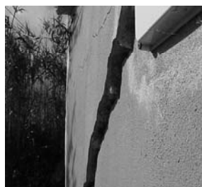
Fig. 19.14. 45° crack in the main façade caused by the displacements of the end wall
