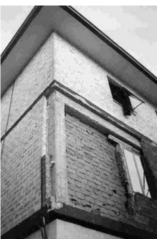
Fig. 16.6. An example of restricted use building
