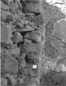
Fig. 19.7. Masonry of irregular stones
