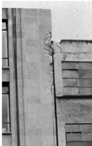
Fig. 13.4. Where the joints between buildings are not sufficiently large to allow them to deform freely, it is highly likely that, in the event of an earthquake, they will collide
