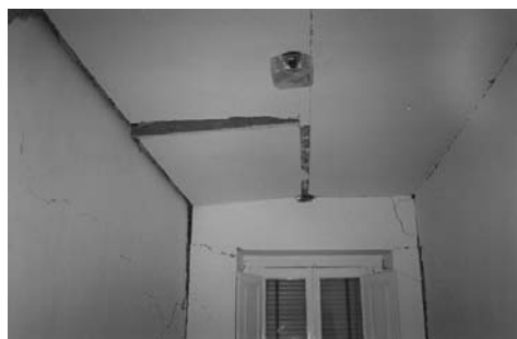
Fig. 16.3. Masonry building. Structural damage
