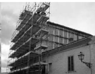
Fig. 16.20. Steel tightening of the church façade (Molise 2002)
