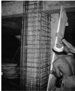
Fig. 19.42. Reinforced concrete encasement technique
