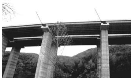
Fig. 14.3. The 1999 Sea of Marmara earthquake. Effects of surface faulting (see the arrows) on the viaduct, near Düzce, part of TEM (Trans-European Motorway). Courtesy of Prof. Polat Gulkan
