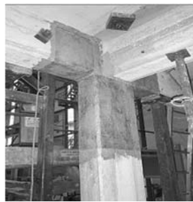
Fig. 19.41. FRP jacketing technique
