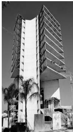
Fig. 13.6. CUBE tower in high seismicity area showing strong discontinuities and long cantilevers (The structural design was done by L. Bozzo)
