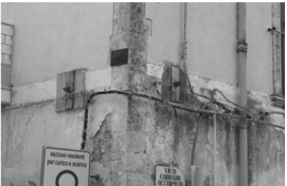
Fig. 19.46. Corner wall confinement with steel plates
