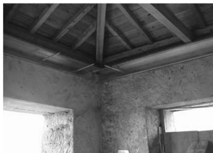
Fig. 19.35. Angle plate supporting the roof braces
