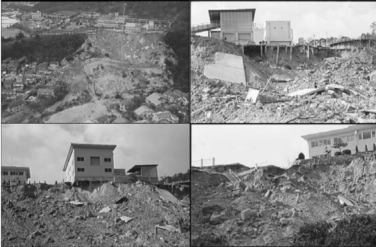
Fig. 4.4. Large landslide in Kobe, Japan caused by the 1995 Hyogoken-Nanbu earthquake, causing the destruction of a large number of houses located on the slopes
