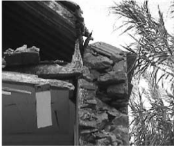
Fig. 19.8. Double-wall masonry
