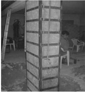
Fig. 19.44. Steel jacketing technique
