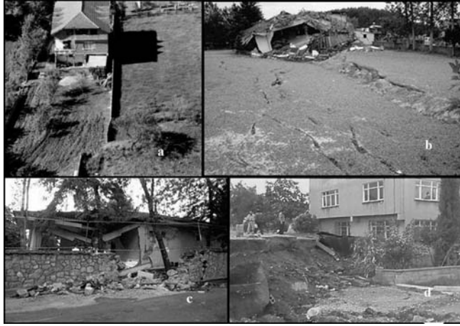
Fig. 4.1. Effects of fault rupture on buildings
