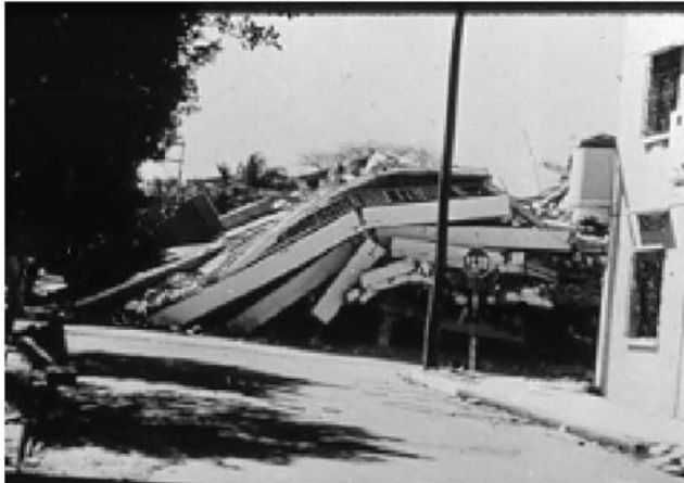
Fig. 13.5. Due to a lack of ductility, structures with slabs as ceilings normally provide unsatisfactory responses
