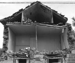
Fig. 19.9. Aspect of the building's interior
