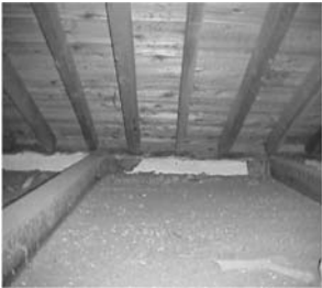
Fig. 19.10. Structural roof solution ("scissor" roof)
