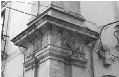
Fig. 19.45. Application of steel forks on the capital
