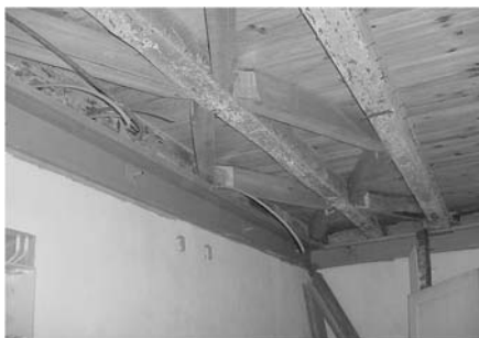
Fig. 19.36. Detail showing the brace support and the angle plate's connection to the wall
