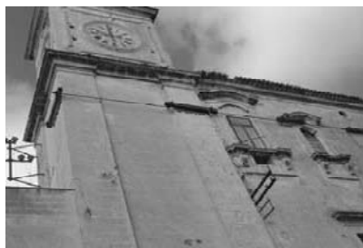
Fig. 19.47. Wall confinement with steel plates and bars
