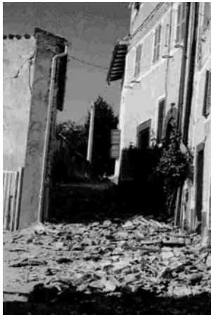
Fig. 16.4. Masonry Building. Non- structural damage
