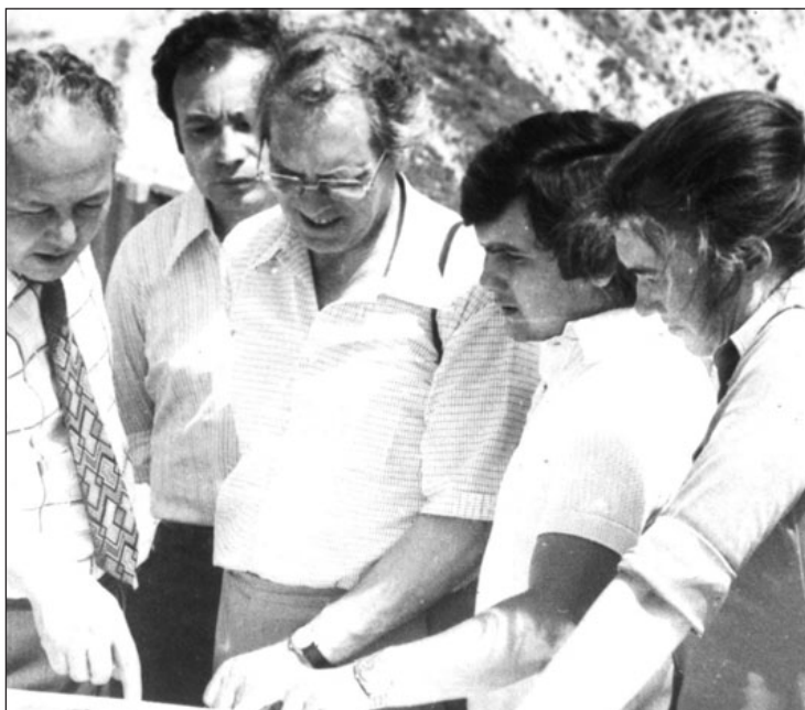
Fig 5. The dam Medeo, Alma-Ata, 1976, R. Wolters in centre discussing materials of "Kazglavselezachita"
