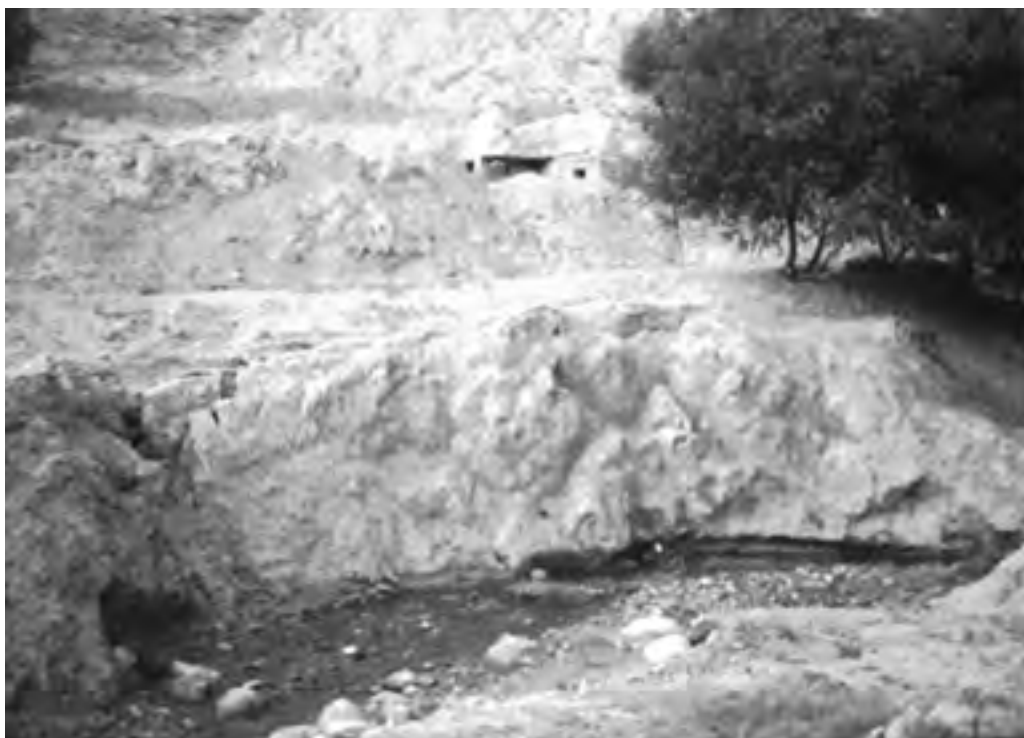
Figure 6.5. Dwelling destroying in Mailuu-Suu river shore
