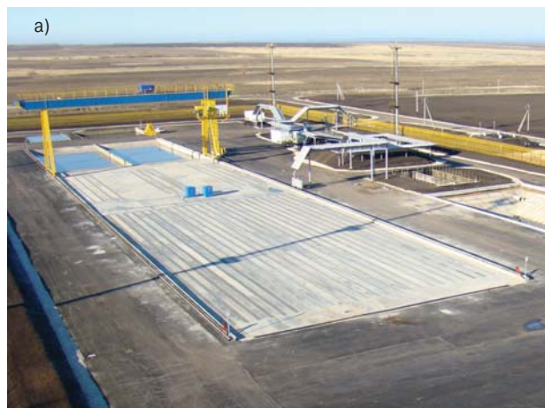
Fig. 4. General view and system of aeration of the complex of biothermal treatment at the Mikhailovsky-Kokhanskoye deposit of Samaraneftgaz OJSC: a – a general view of the complex with air channels; b – blower for stack aeration; c – aeration channels
